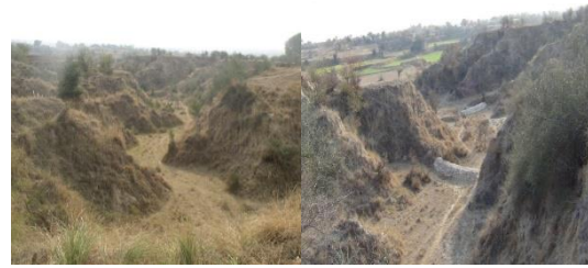
Fig. 2 Gully development with check dams
