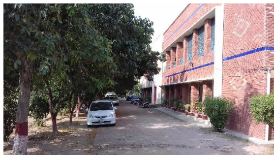
Figure 1: Office of the Sugarcane Research Institute, Faisalabad
